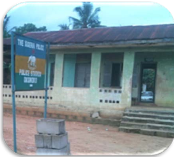
Plate1: Showing the presence of a dilapidated Police Post In the study area Source: Authors' field trip, 2015
